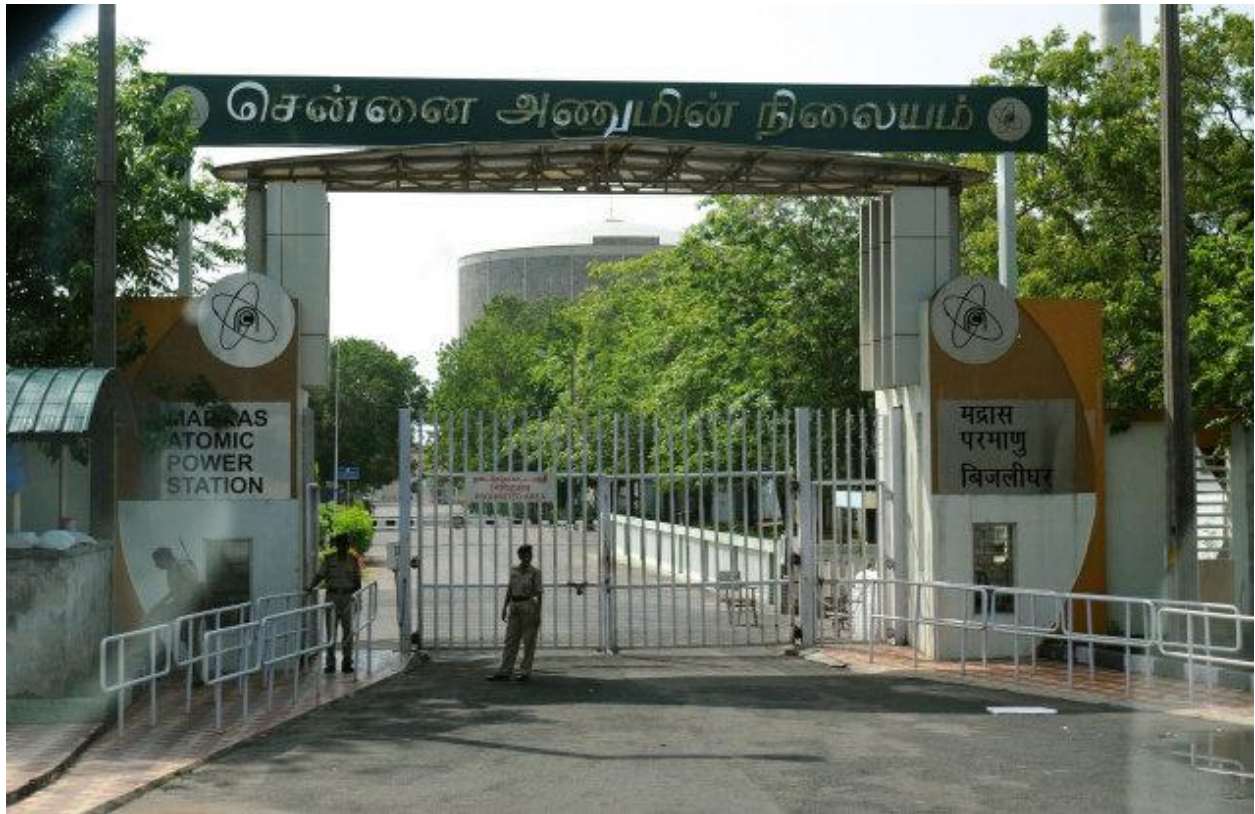
Figure 11 - CISF guards at a gated entrance to the Madras Atomic Power Station, which is located at Kalpakkam, about 80 kilometers south of Chennai. (Photograph courtesy of the Department of Atomic Energy, Government of India)
